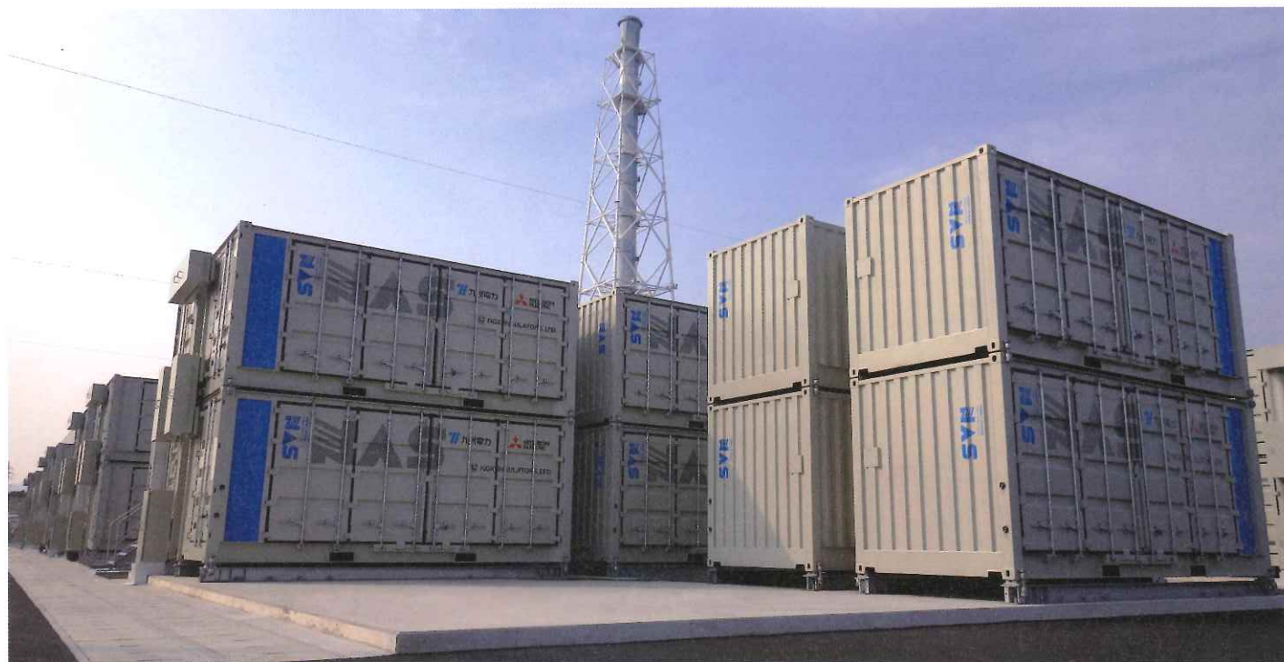
Container-type NAS battery ordered by Mitsubishi Electric Corporation and delivered to the Buzen Substation of Kyushu Electric Power Co., Inc.
