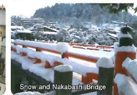
Snow and Nakabashi Bridge
